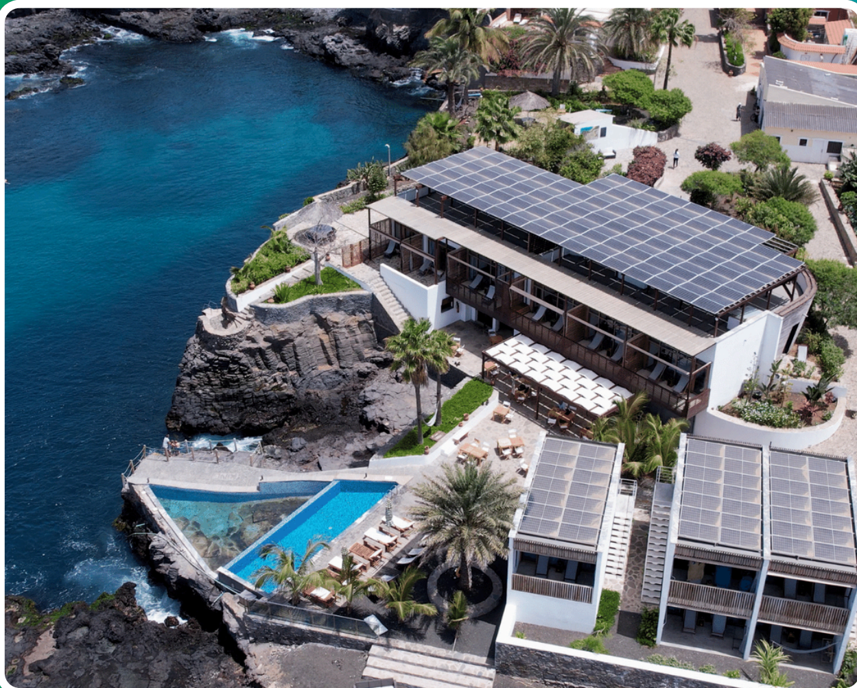
VISTA AÉREA DO HOTEL KING FISHER VILLAGE COM OS PAINÉIS INSTALADOS NO TELHADO DO EMPREEDIMENTO TURÍSTICO. AERIAL VIEW OF THE KING FISHER VILLAGE HOTEL WITH THE PANELS INSTALLED ON THE ROOF OF THE TOURIST VILLAGE
