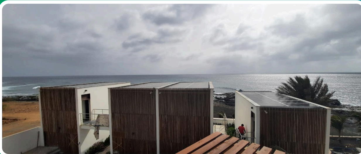
SISTEMA SOLAR FV INSTALADO NO TELHADO SOLAR PV SYSTEM INSTALLED ON THE ROOF
