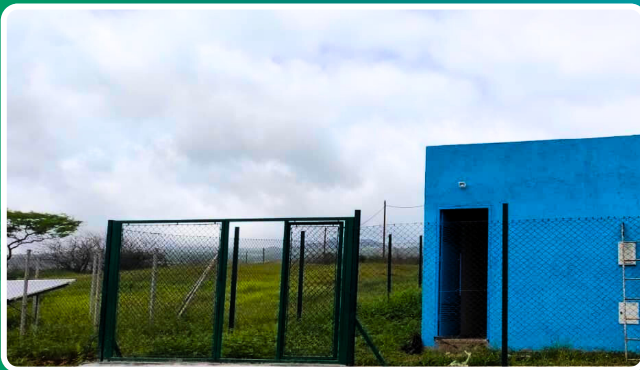
ENTRADA NA INFRAESTRUTURA DO FURO FBE-58 DE JOÃO VARELA THE ENTRANCE TO JOÃO VARELA'S FBE-58 DEBOREHOLE INFRASTRUCTURE
